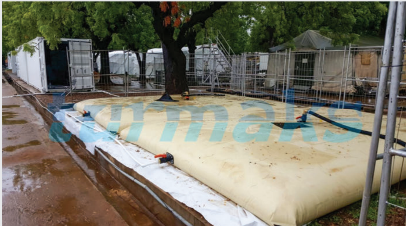
WATER BLADDER TANK
